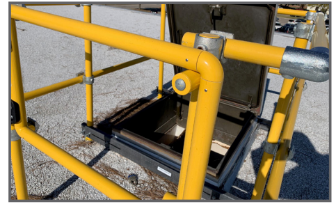
Self-closing gate prevents accidental entry.
