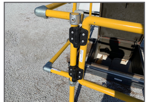
Rugged hinges allow gate tension adjustment.
